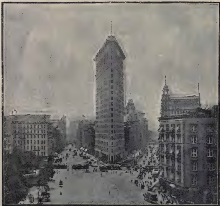
FIG. 156—Flatiron Building at the junction of Broadway, Fifth Avenue and Twenty-Third Street, the heart of New York. This building is twenty-one stories high
